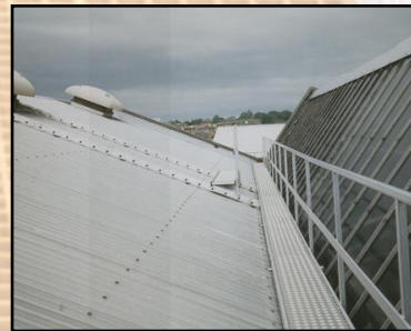
Alloy framed walkway fitted with solid alloy 5 bar tread plate decking removable for gutter cleaning.
