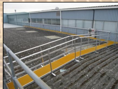
Alloy framed walkway with GRP decking fitted to inclined asbestos sheeting
